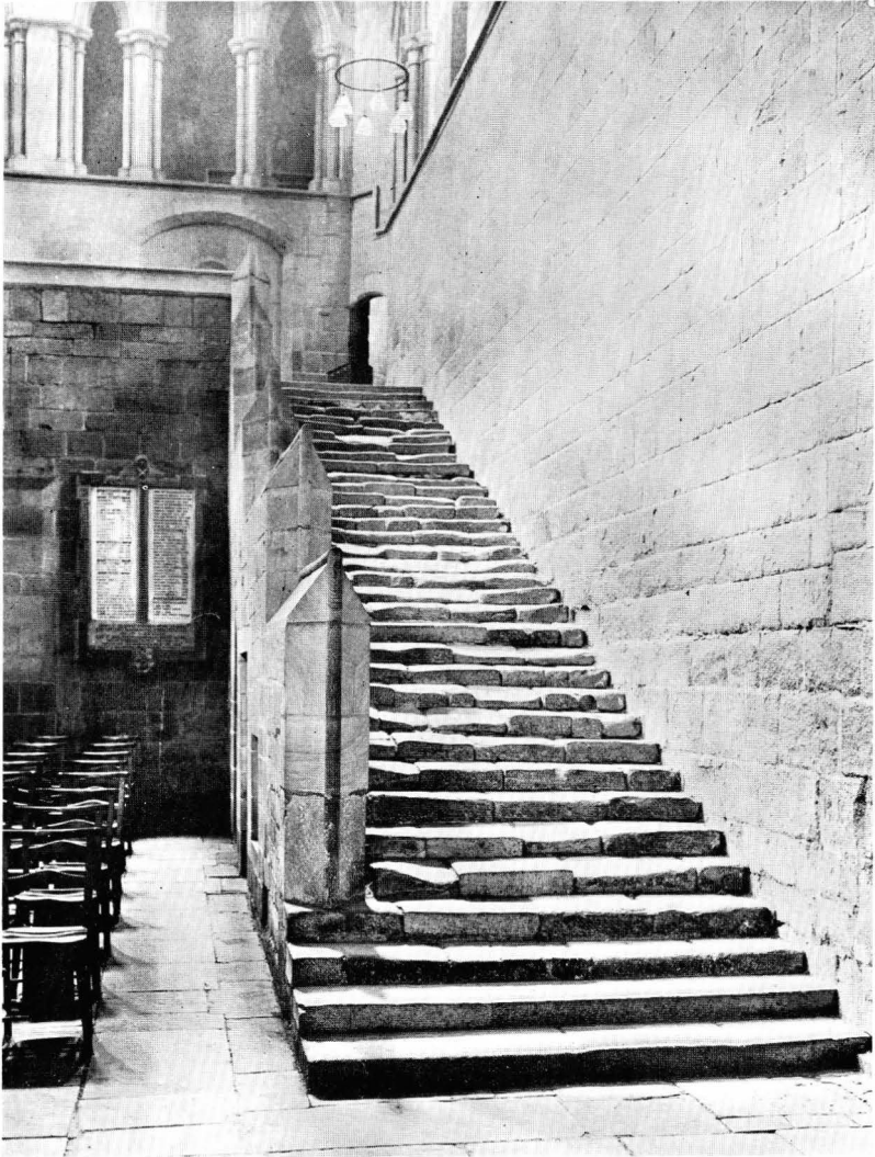
FIG. 44.—HEXHAM PRIORY, NORTHUMBERLAND. NIGHT STAIRS.
