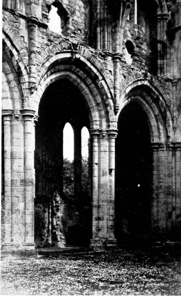
FIG. 17.—NETLEY ABBEY, HANTS. SOUTH TRANSEPTAL CHAPELS.
