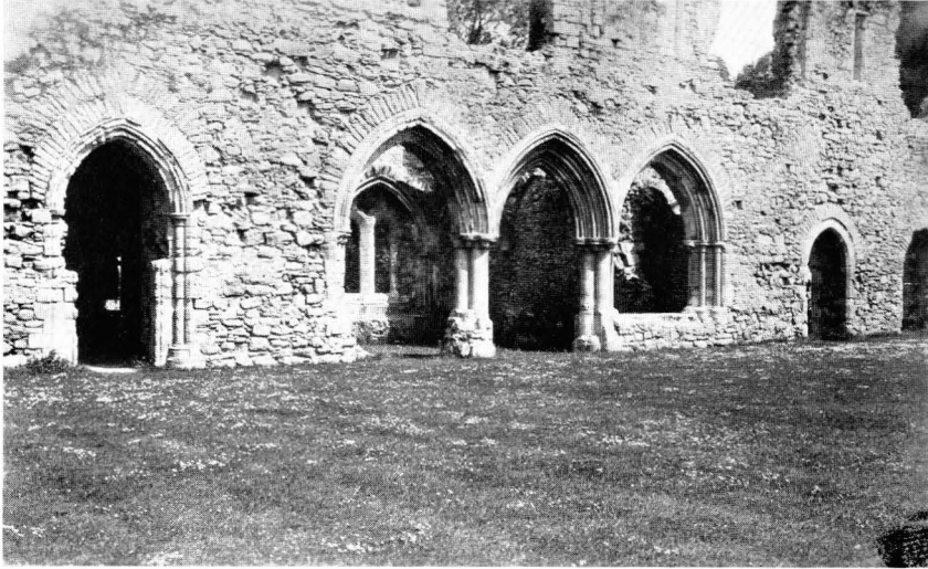
FIG. 46.—NETLEY ABBEY, HANTS. EAST RANGE OF CLOISTER. Showing entrance to Sacristy, Chapter-house, Slype, and Dorter windows over.
