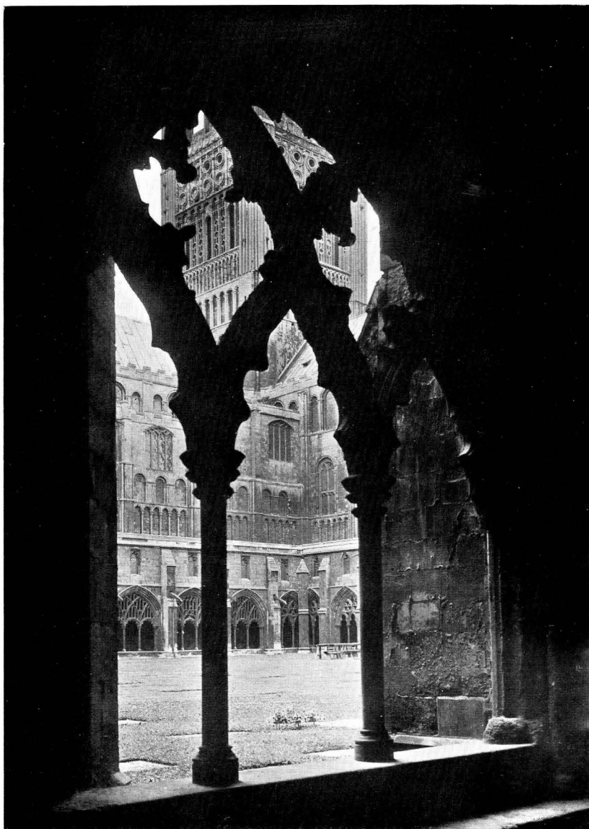
FIG. 35.—NORWICH CATHEDRAL PRIORY. CLOISTER AND CHURCH.
