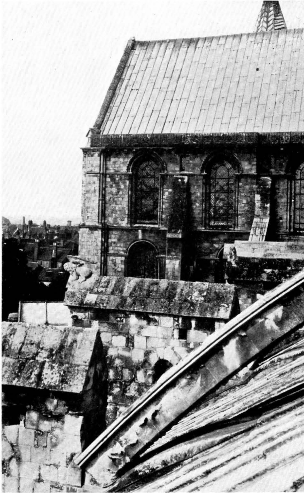
FIG. 32.—CANTERBURY CATHEDRAL. FLYING BUTTRESS TO QUIRE.
