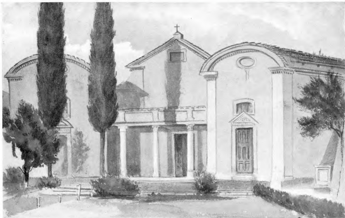
THE THREE CHAPELS OF ST. ANDREW, SANTA SILVIA, AND SANTA BARBARA, ORIGINALLY BUILT BY SAINT GREGORY, AND REBUILT IN THE SEVENTEENTH CENTURY.
