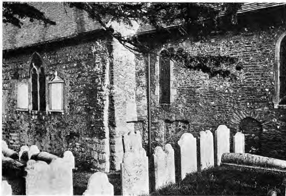
REMAINS OF SAXON WORK AT ST. MARTIN'S, CANTERBURY.
